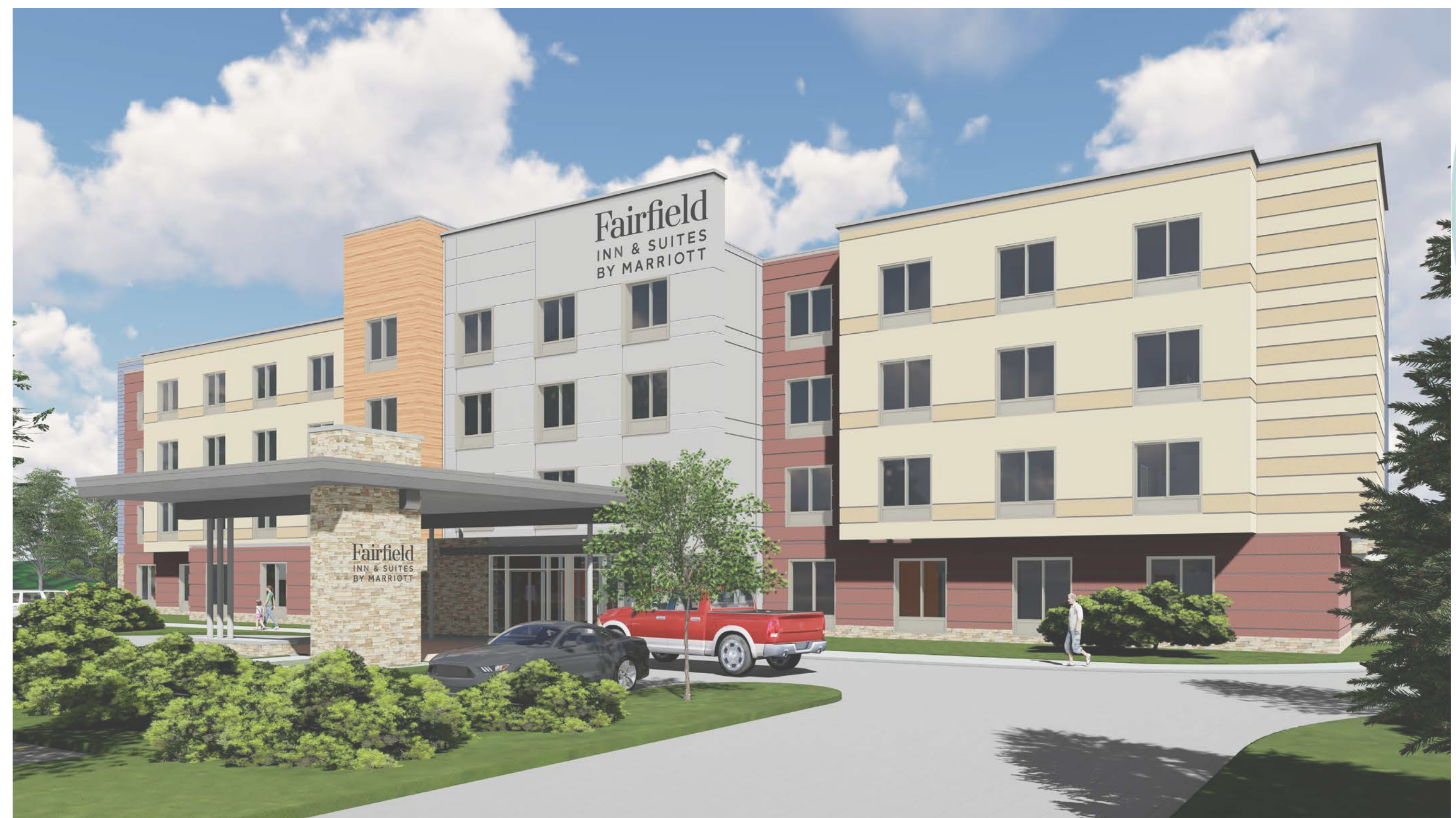
VIEW LOOKING FROM SOUTH WEST
