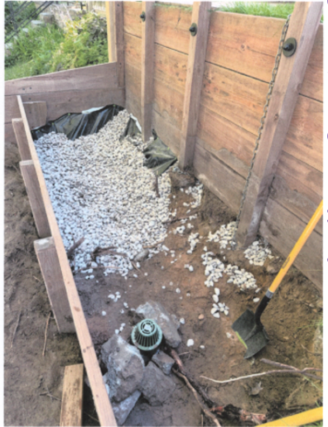
12) Outlet Fix. 70% Drain Stone
