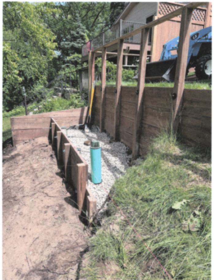
12) Outlet Fix. 70% Drain Stone
