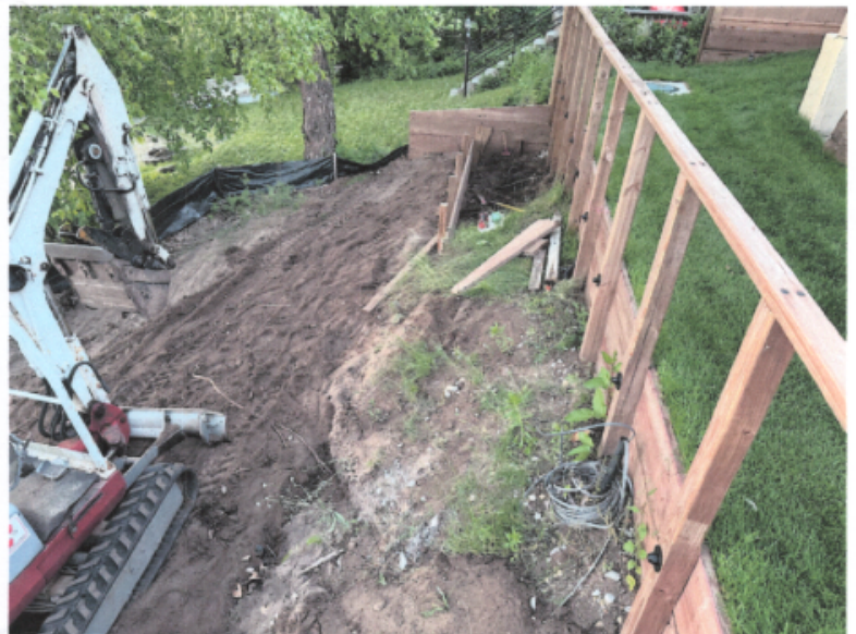
8) Backfill over outlet pipe
